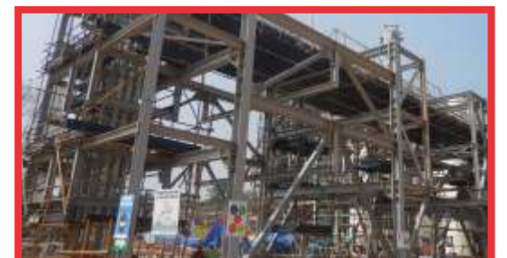
Fabricated Structural Steel
