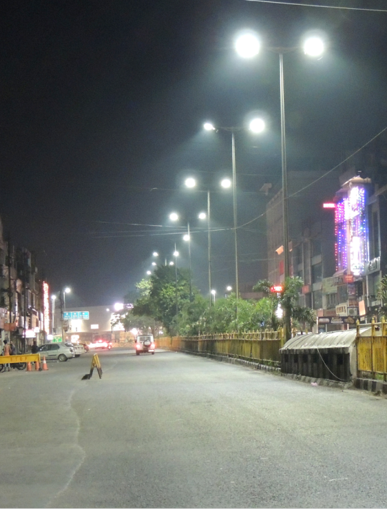
New Market Road BRTS
